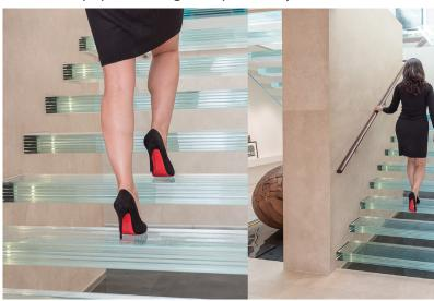
PROJECT DETAILS: Collection: Josiah J Series: Glass Sandpaper Treads Texture/Walking Surface: Glass Sandpaper Glass: Low Iron Thickness : 3.3" (84mm) Dimensions: 62" x 14" Treads, 62" x 62" Landings Designer: Hollingsworth Architecture, West Vancouver Installer: Horizon Glass
